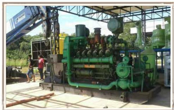
Gasification technology is the use of biomass fuel to burn in a specially designed furnace which is called as Gasifier stove, it will control the amount of air entering the furnace in lesser volume than usual to force the situation which is called “Incomplete combustion”. Such condition will cause the heat inside the stove approximately 1100 degrees Celsius and there are five types of gas occurred:
