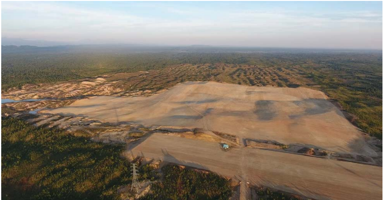
Figure 2-6: Bird's-eye view of Project Minbu
